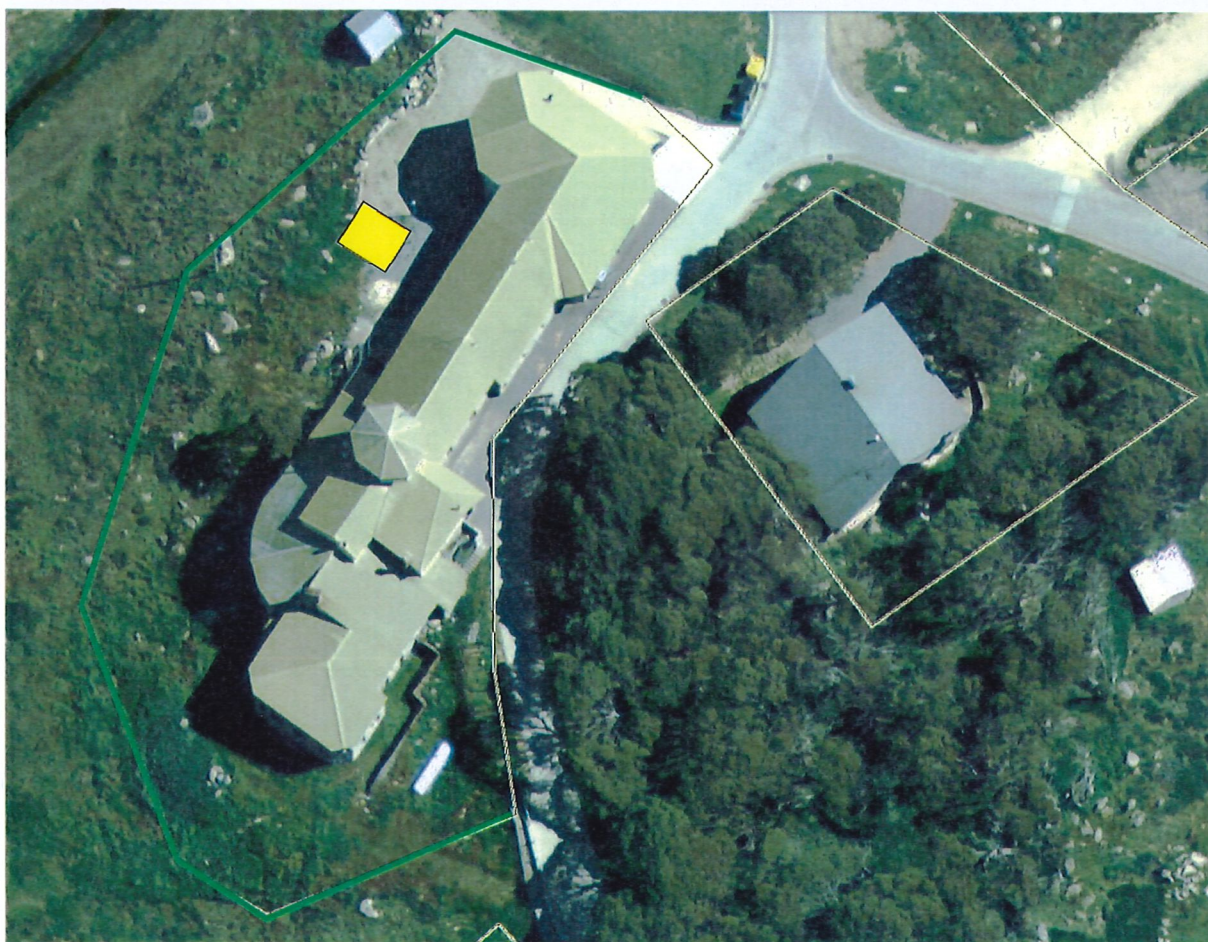
SEDIMENTATION CONTROL, WASTE MATERIAL STORAGE ZONE
