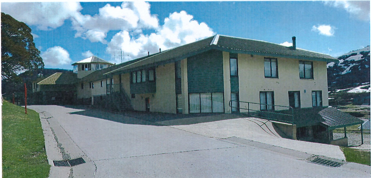
South and East Elevations
